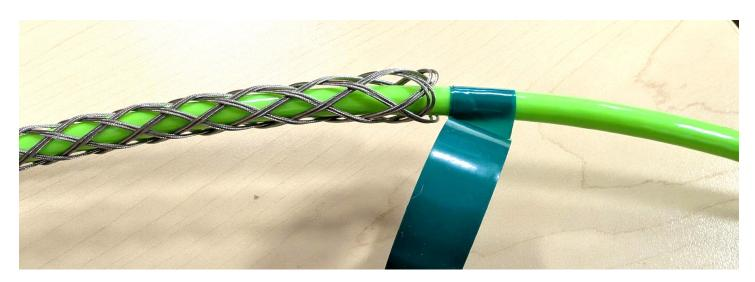
• Continue to wrap the tape over the last 25mm of the tail, and then continue to wrap back down onto the cable.
